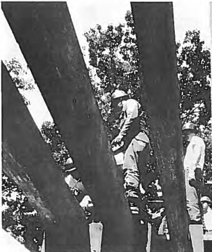
Engineer "Pioneers" of the 3rd Brigade build a bridge.
