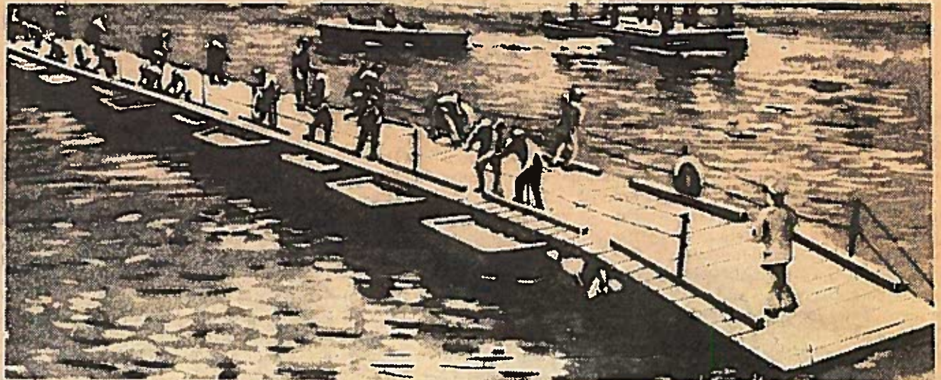
Soviet Troops Emplace the LPP (Light Pontoon Bridge)
