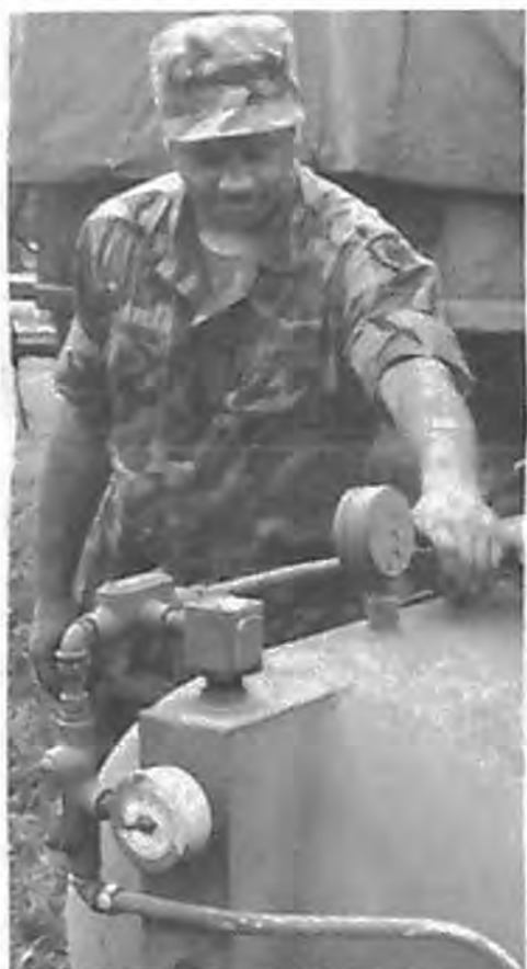
Spc. Benjamin Robinson checks a valve on a portable hot water boiler during a shower point mission at Constantia, N.Y. (Photo by Terry Brown)
