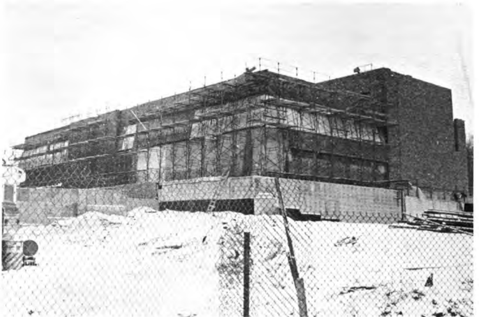
Above photo shows construction of the new Fisher library.
