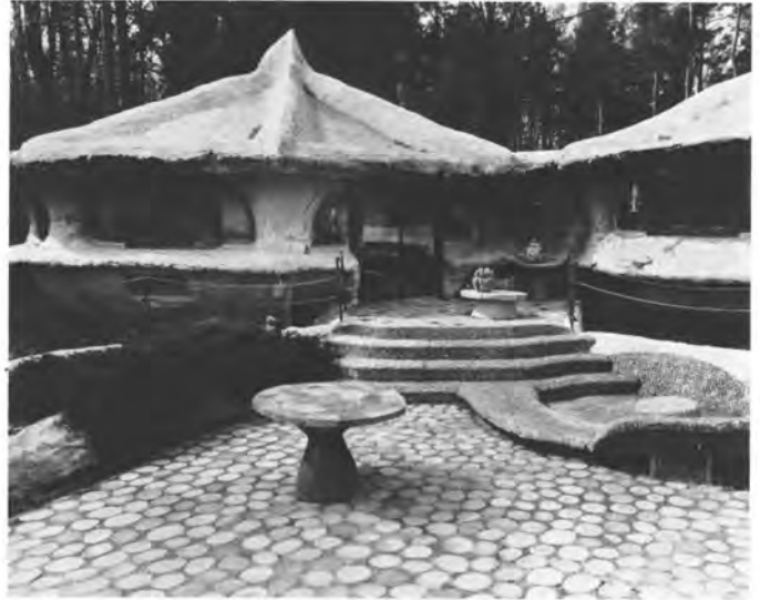
CELEBRATED STRUCTURE near the Basin is the "mushroom house" built by Mr. and Mrs. Robert Antell, Park Rd. For those within, it gives the impression of floating amid treetops.
