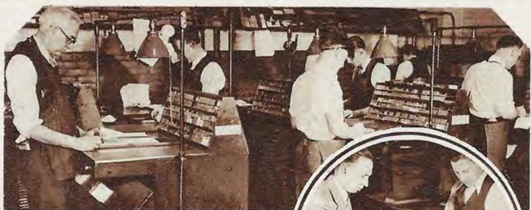
Advertisements are assembled in the ad alley, a section of which is above. Make-up of pages under direction of an editor is the last operation before stereotyping
