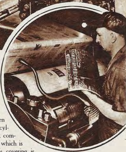
Each plate cylinder like the one shown in the detail at the right carries eight page plates, making 16 pages to the press unit. The pressman in the picture is placing a page one plate on the cylinder.
