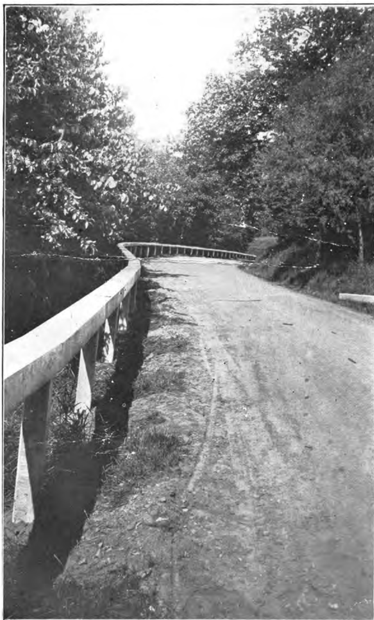
CONCRETE GUARD RAIL ON ATLANTIC AVENUE DUGWAY Making a Beautiful Highway Wider and More Attractive
