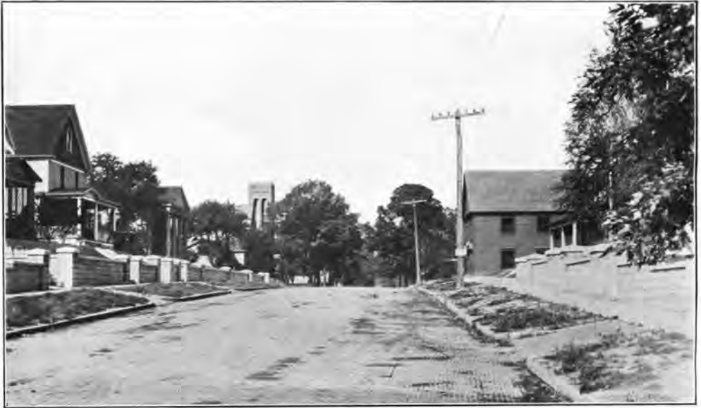
STUTSON ST. APPROACH TO CHARLOTTE BRIDGE, ROCHESTER Showing McClintock Cube Pavement Entrance to Lake Shore Boulevard, made possible by recently adopted constitutional proposition
