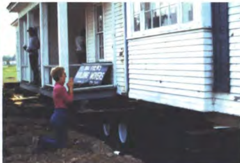
Gretchen Howe says a prayer that her family home will arrive safely on its new site just before the move begins.
