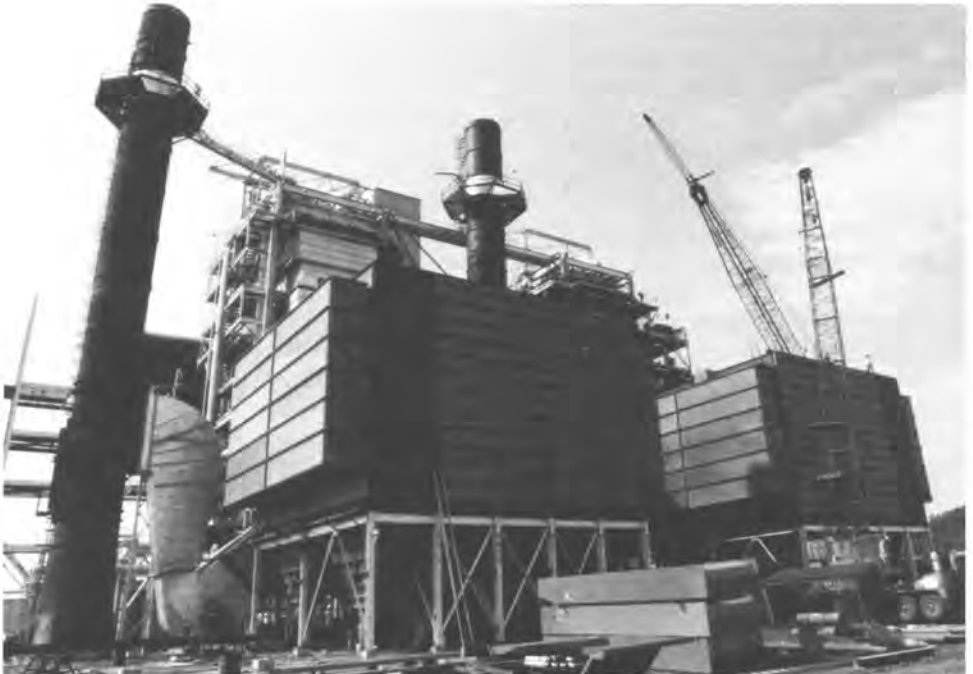
Conversion of boiler systems from natural gas to coal energy is among several major projects being completed at Eastman Chemicals Division plants.
