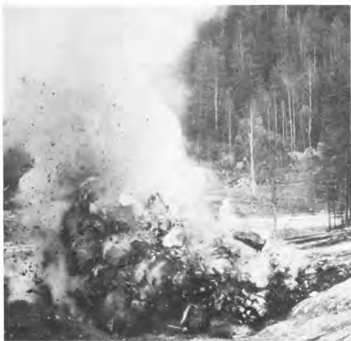
Ground breaking started at 3 p.m. on Oct. 26 with this blast of rock.
