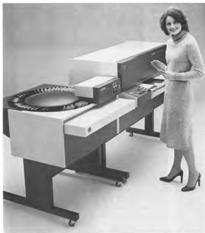
Designed for operator convenience and efficiency, the new Kodak Ektafiche collator, used with the Kodak Ektafiche duplicator, substantially improves the effectiveness and productivity of in-house microfiche operations. The collator and duplicator both meet world safety and electrical requirements.
