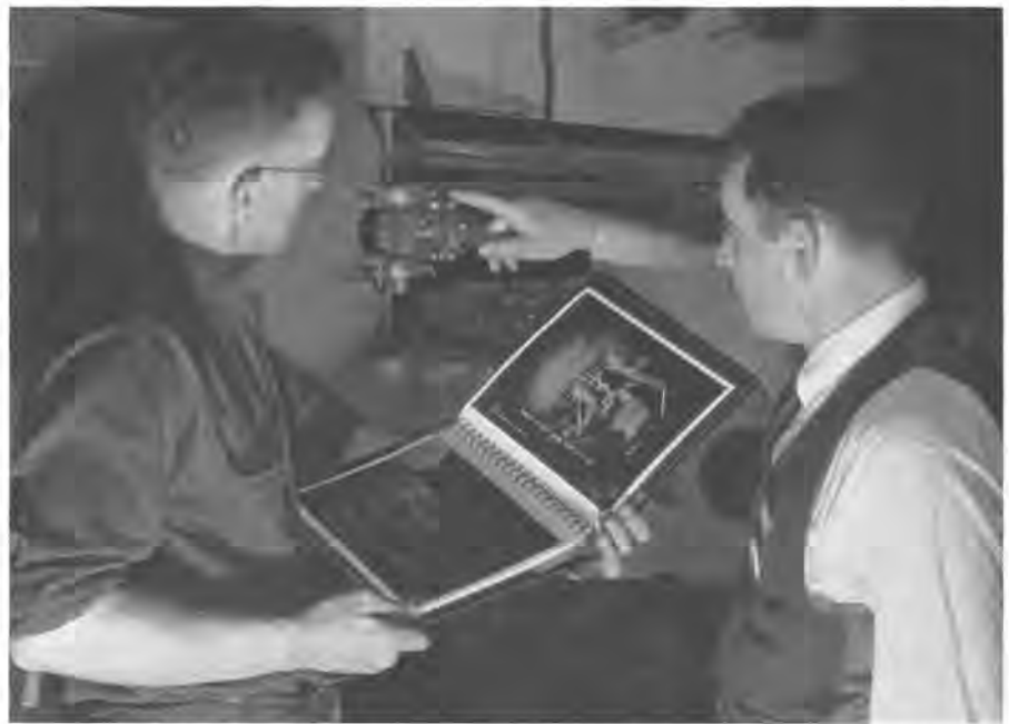
At the Bell Aircraft plant in Buffalo, an employee receives instruction on the job from his supervisor. Each step of his work is checked against one of a series of photographs bound in a manual
