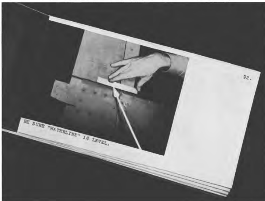
One type of visual instruction manual at Bell Aircraft is shown here. Each succeeding step in the installation of the hood over the Airacobra's cockpit is here outlined in a series of photographs
