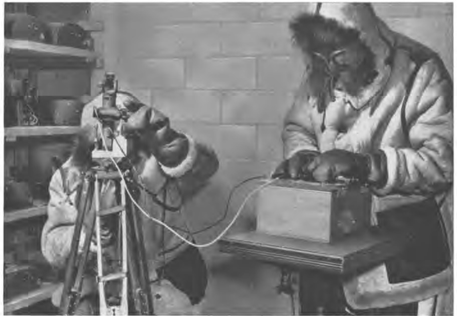
The Kodak-made M-12 panoramic telescope, an important instrument of war, is brought to high-altitude temperature in the Arctic Chamber. Thermocouple wires, leading from the telescope to a testing instrument, measure the below-zero temperature of the room
