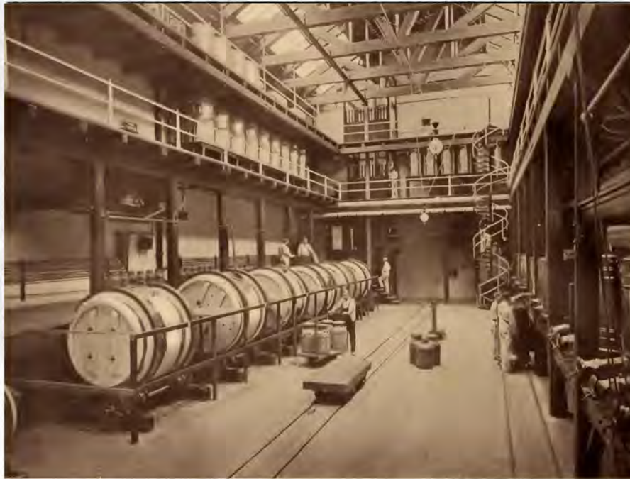
The Dope Building, Kodak Park, Where the Materials for the Transparent Film Base are Mixed and Clarified.
