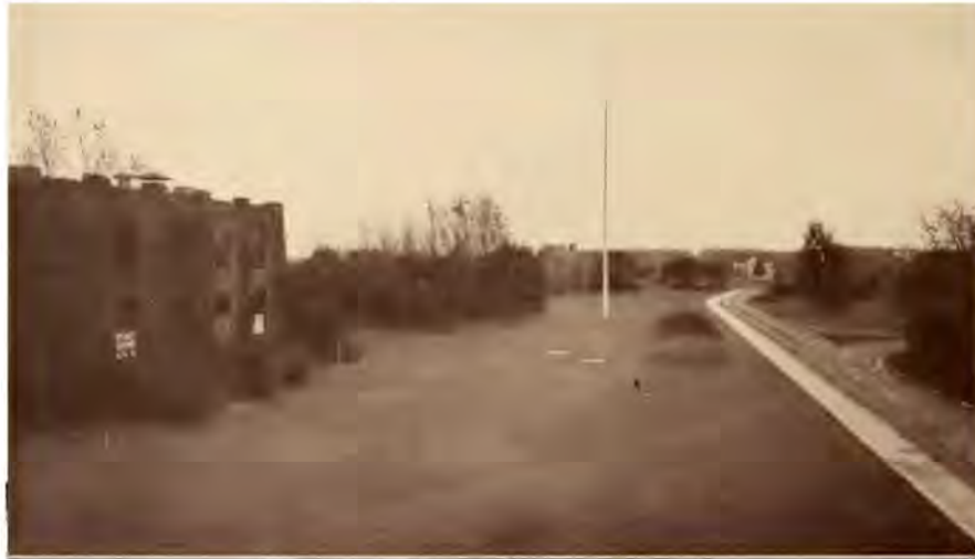
Looking Toward the Boulevard From Kodak Park Office.
