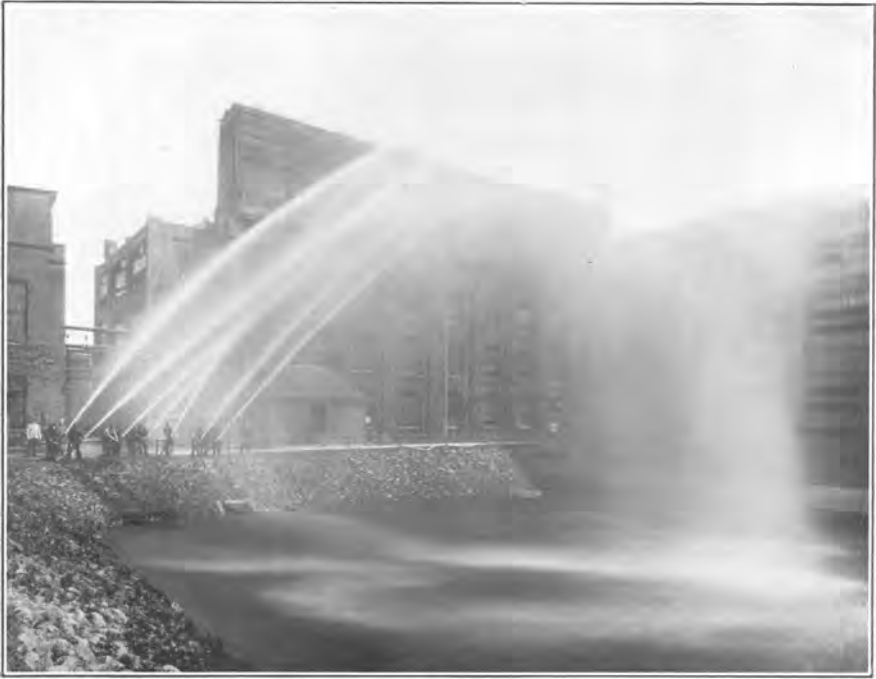
Test of Fire Mains
