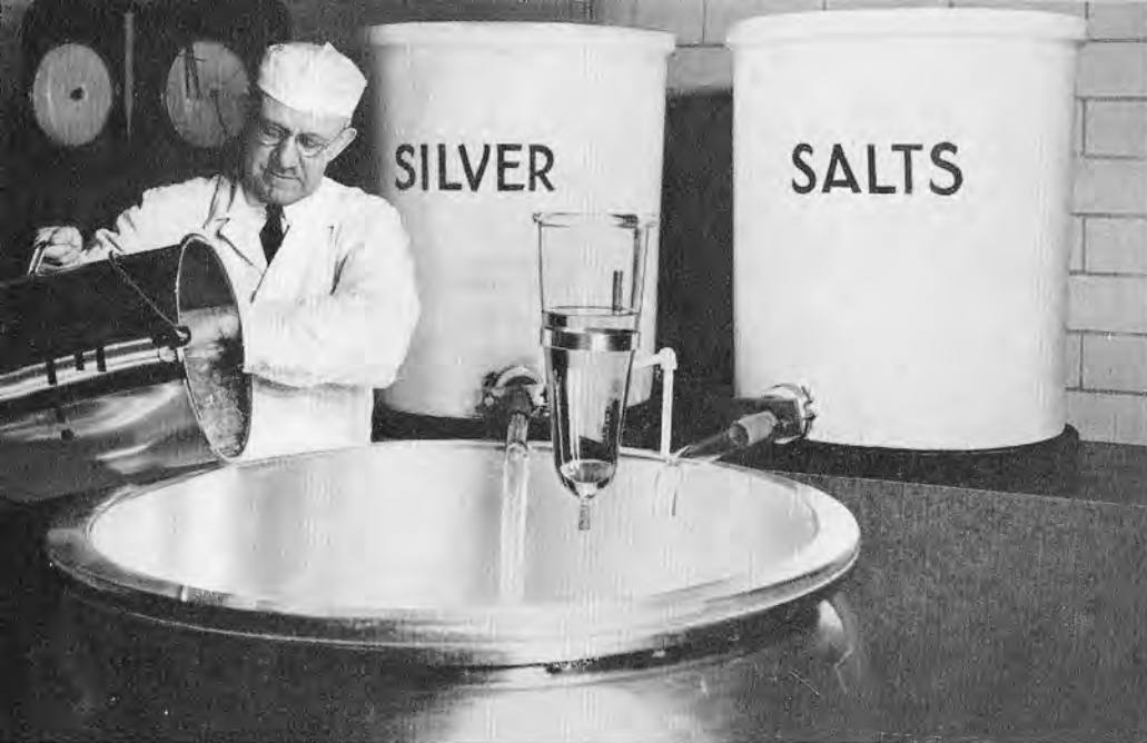
Combining ingredients for photographic emulsion.
