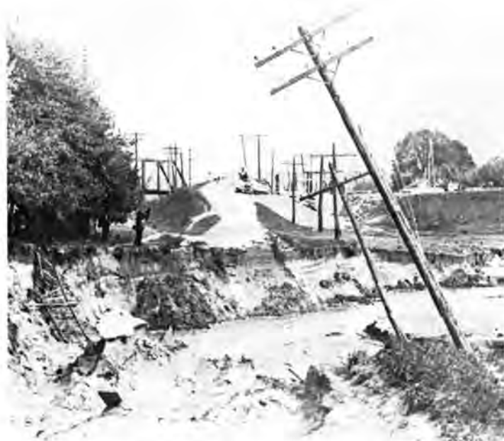
A look at the Bushnell's Basin canal break of 1908, looking east at the Marsh Rd. bridge.
