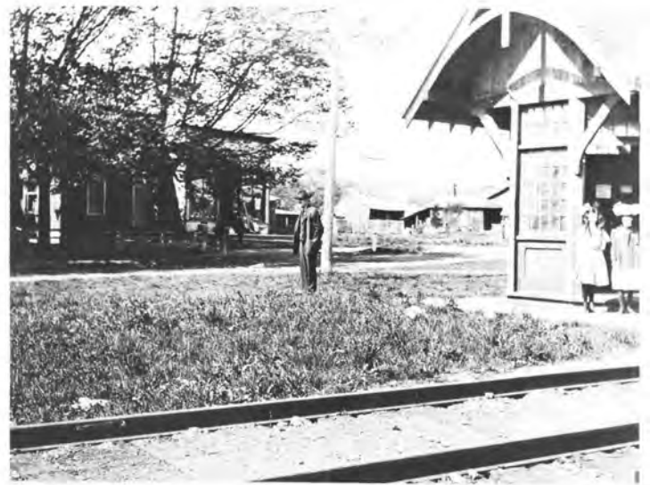
This gentleman and the two girls are waiting for the next train to Rochester at the Egypt train station.
