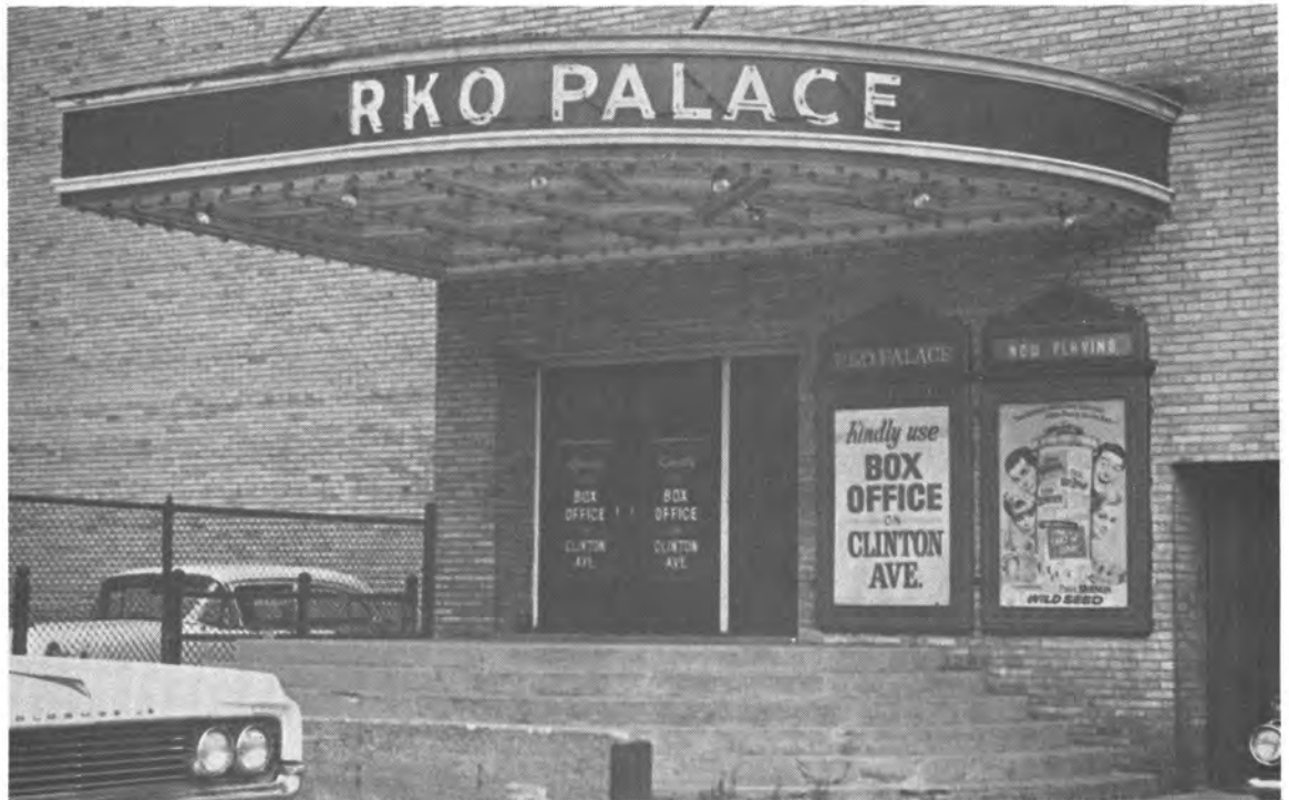
Side entrance showing box office
