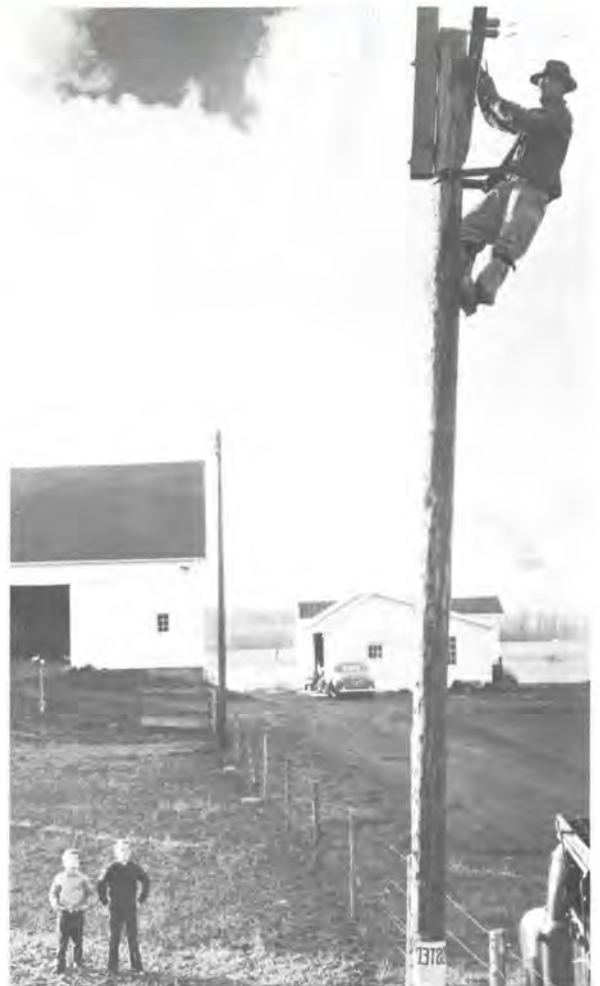
Rochester Telephone Installer in rural setting.
