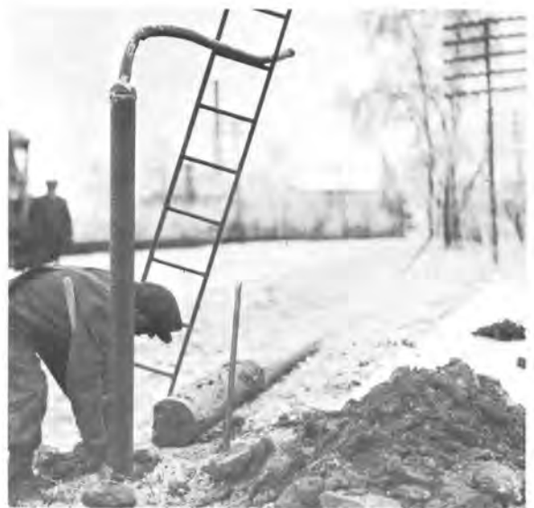
Cable Repairman works to repair damage after sleet storm in 1929.
