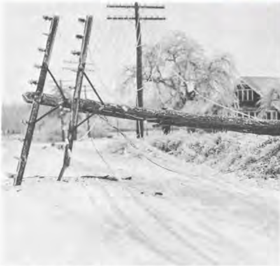
Pole felled in West Chili by 1929 sleet storm.
