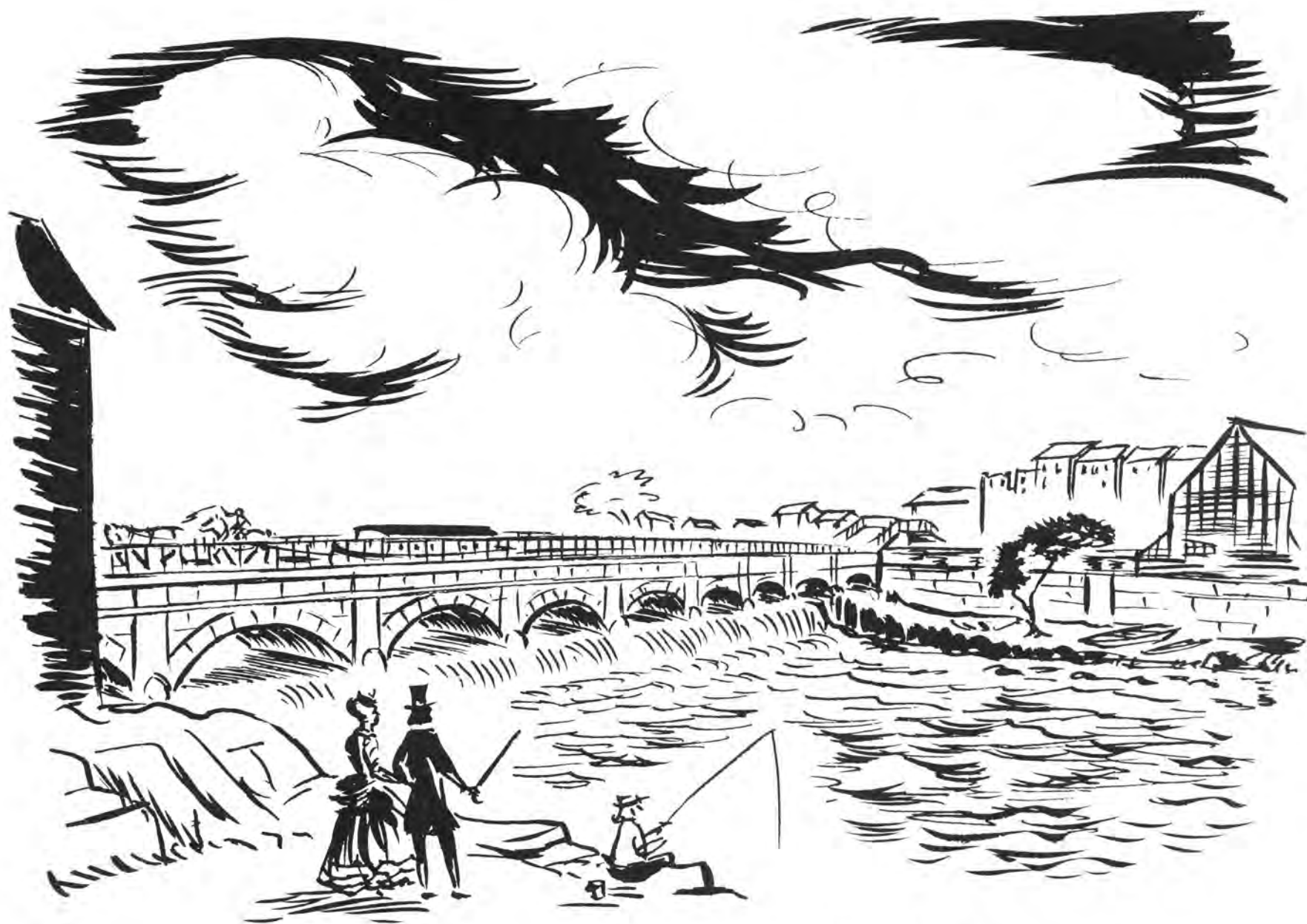
An Aqueduct of the Erie Canal Crossing the Genesee River in Rochester
