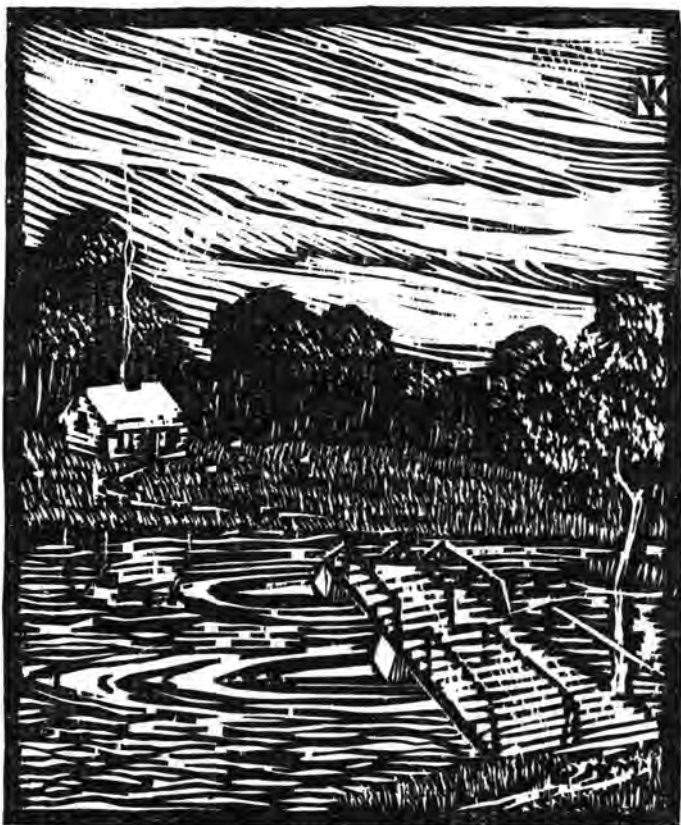
THE FIRST MAIN BRIDGE (BEFORE COMPLETION)
