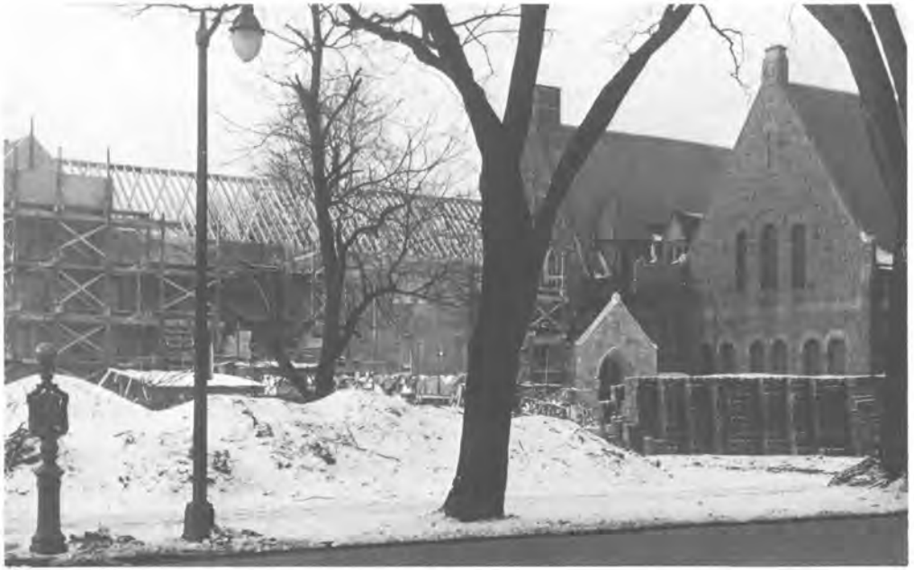
The present Chapel and Education Building during construction.
