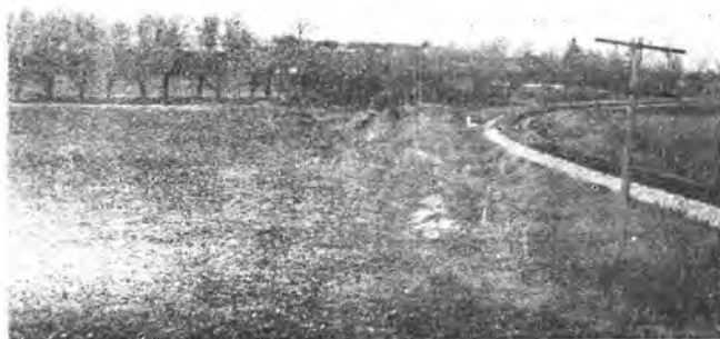
Horse railroad ran thru cut in center and on embankment beyond west of Harbuttsville can still be seen 1973
