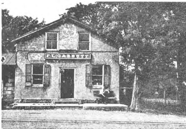
Garbutt Store—Horse railroad passed under original porch at cellar level
