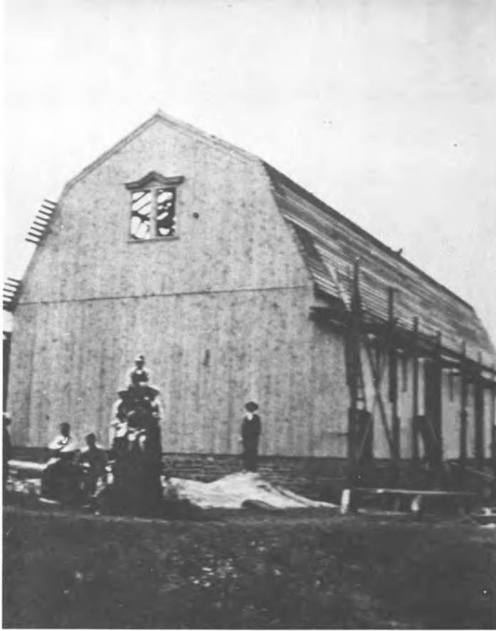
A Wells barn under construction.
