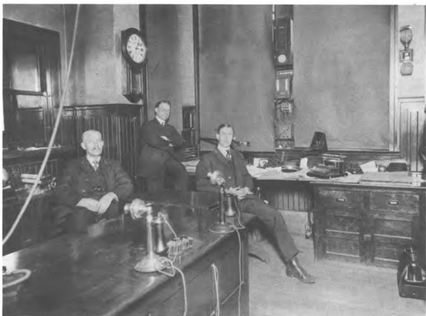
Office Mumford station on Mumford - Caledonia Road. Mr. Hadley behind desk, Mr. James Baldeck sitting at end of desk, an inspector in the background.
