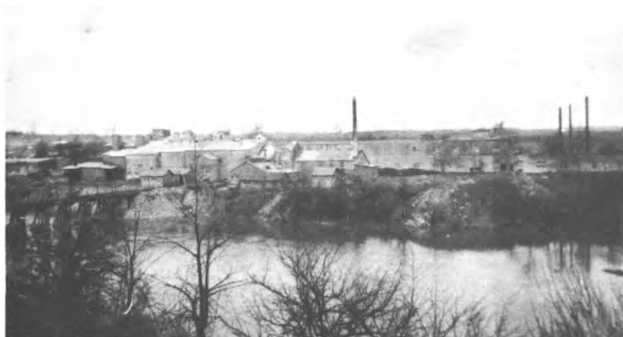
Lycoming Calcining Company. View across the creek showing the Lycoming Mill Bridge.
