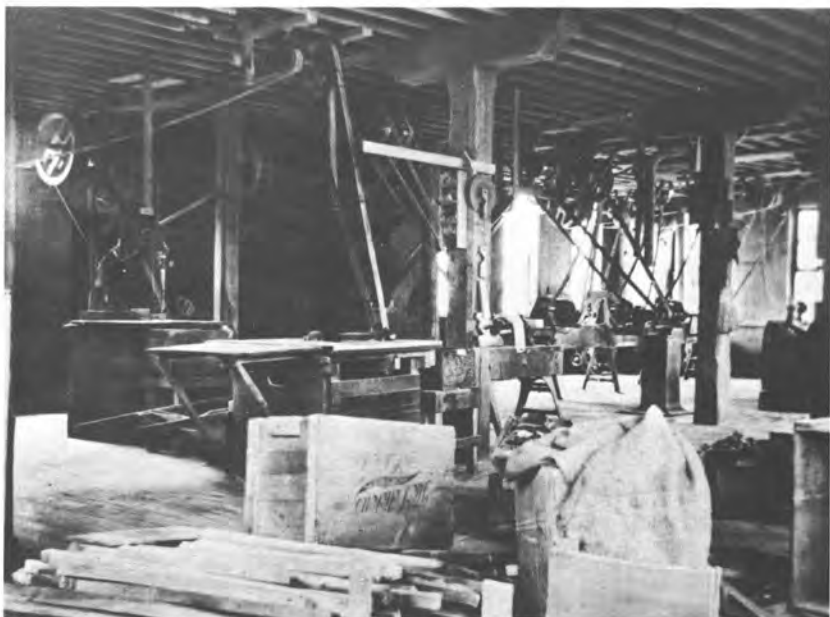
Interior of pipe factory, Mumford, N.Y. Machines used to saw wood into lengths for pipes.
