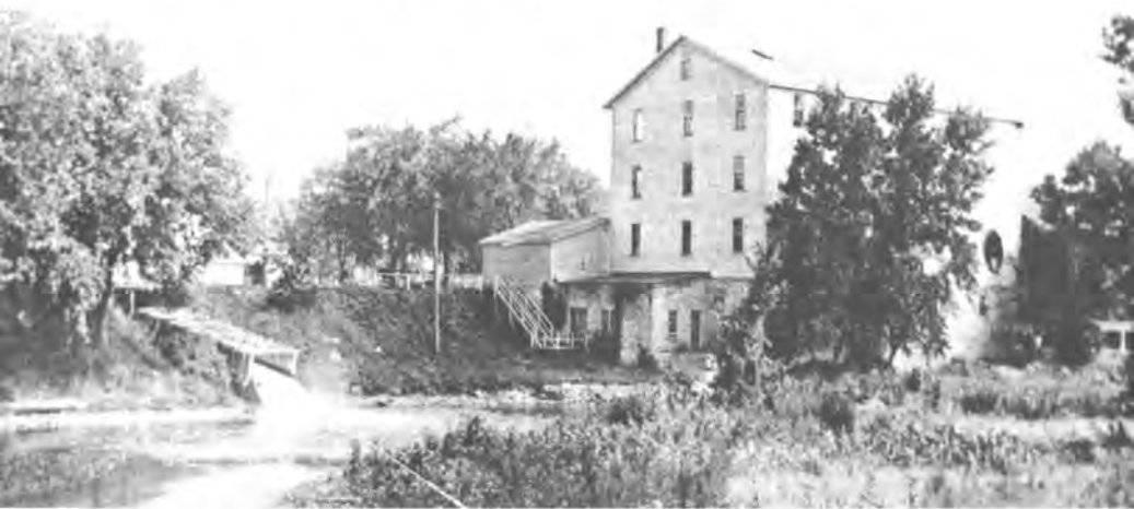
Smith's Mill, later Wheatland Milling and Power Co. Mill, on the south side of Main St., Scottsville, N.Y. Showing the flue on the left, that came down out of the race. On the side of the mill is the electric light plant, built by John T. Wells and sons for the Wheatland Milling and Power Co. Isaac Salyers was the first president, he made application for the purpose of lighting dwellings, streets and stores.
