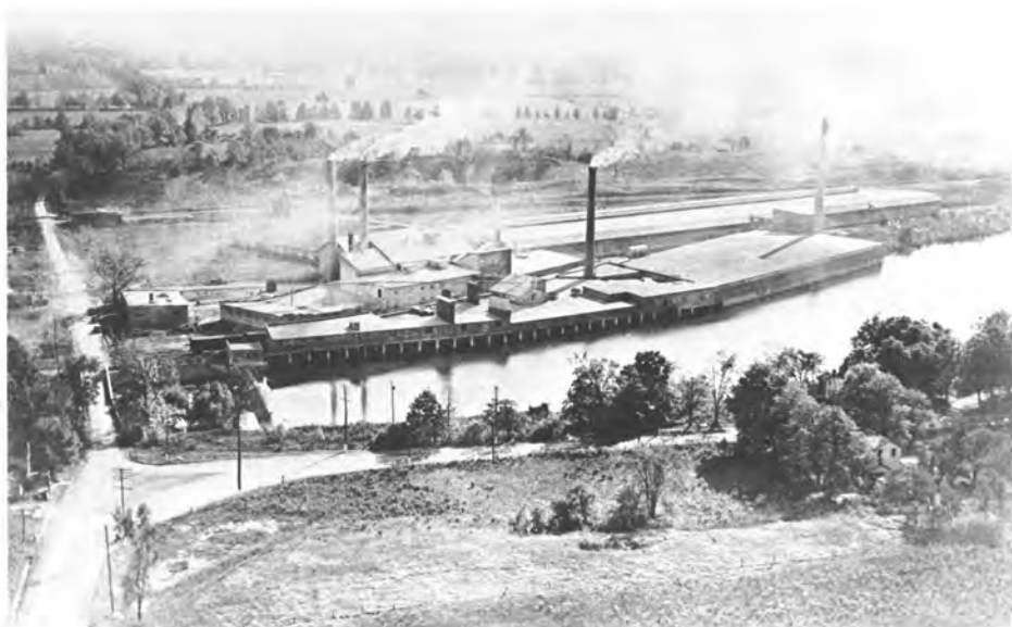
Ebsary Mill, Wheatland Center looking south across Oatka Creek. Mill workers' homes to the right front and the miller's house.
