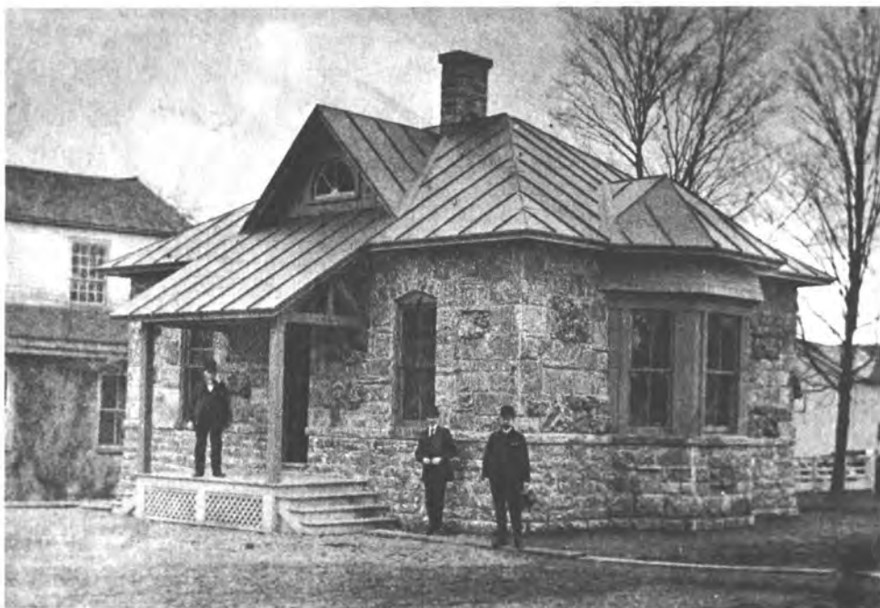
Office of Allen's Woolen Mills. Armstrong Road, Mumford.
