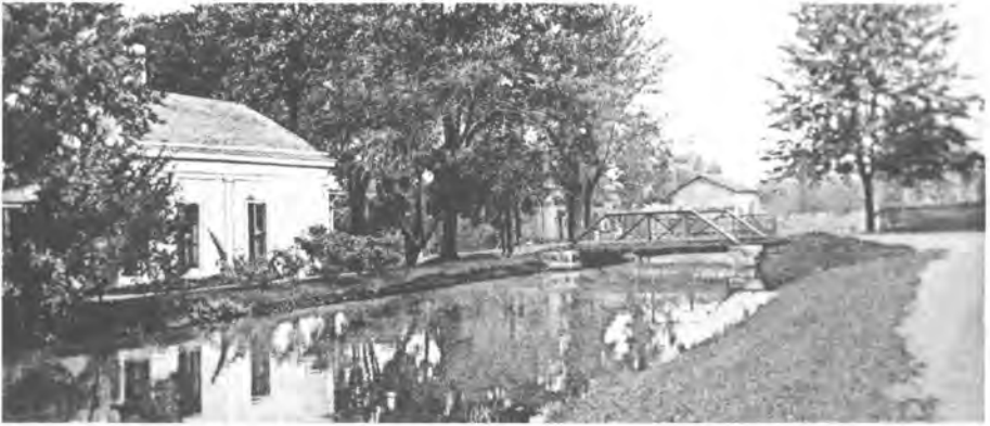
Bridge over the raceway on Main St. In 1826 Abraham Hanford and Powell Carpenter built a dam across the Oatka on Burrell's flats, under the supervision and engineering of Alvin Savage, and constructed a raceway one and a quarter miles in length from the dam to the mill, obtaining a fall of twenty feet and a volume of water with power sufficient to operate two mills.
