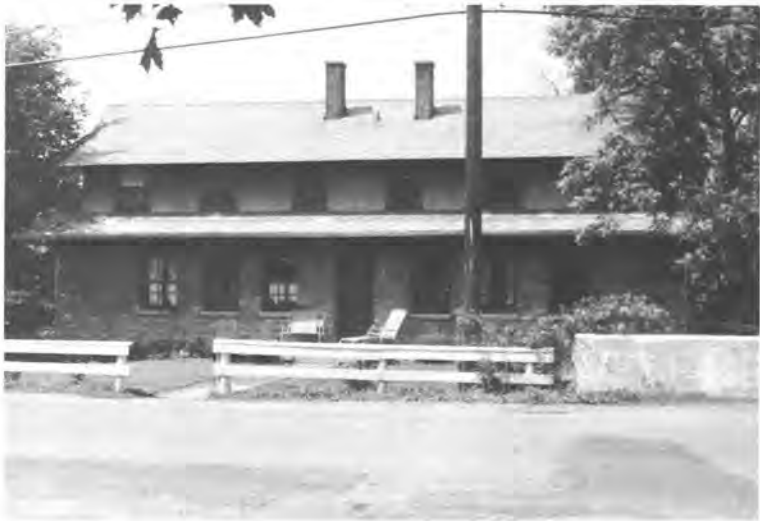
Garbutt Plaster Mill used as a residence for L. H. Gardner, paper mill manager.
